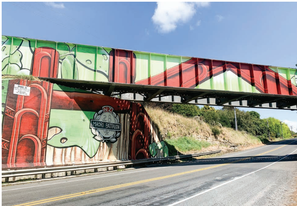
The subway bridge resplendant with its new mural
