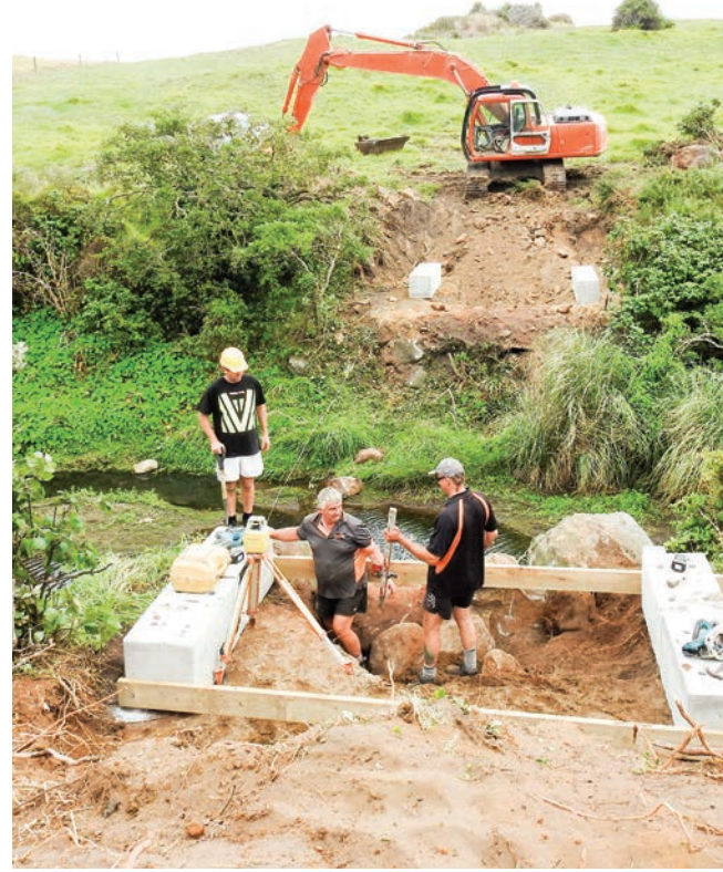
The team at Bridge It NZ get to work.
