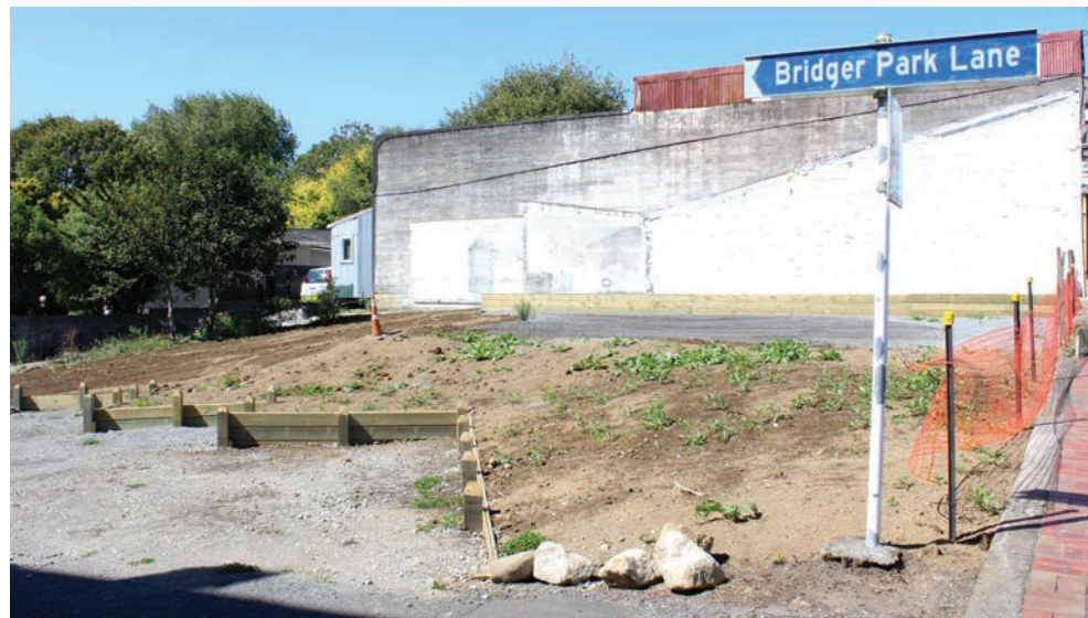
Development of a new entrance to Bridger Park is starting to take shape.
